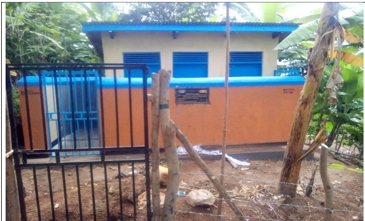
Bunango Rural Growth Centre Composite Latrine completed
