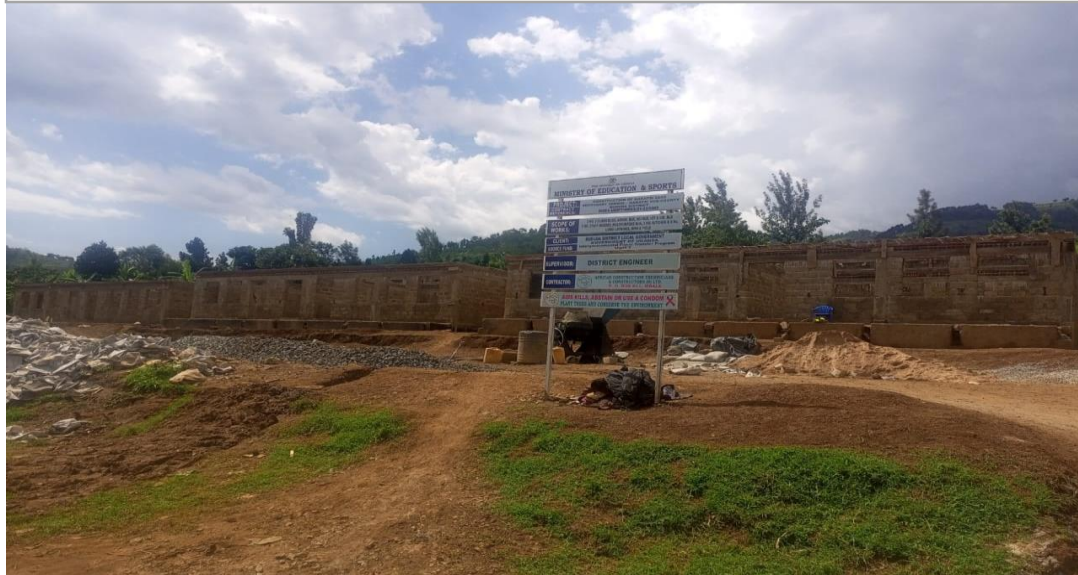
• Nakatsi Seed Secondary School at roofing level
