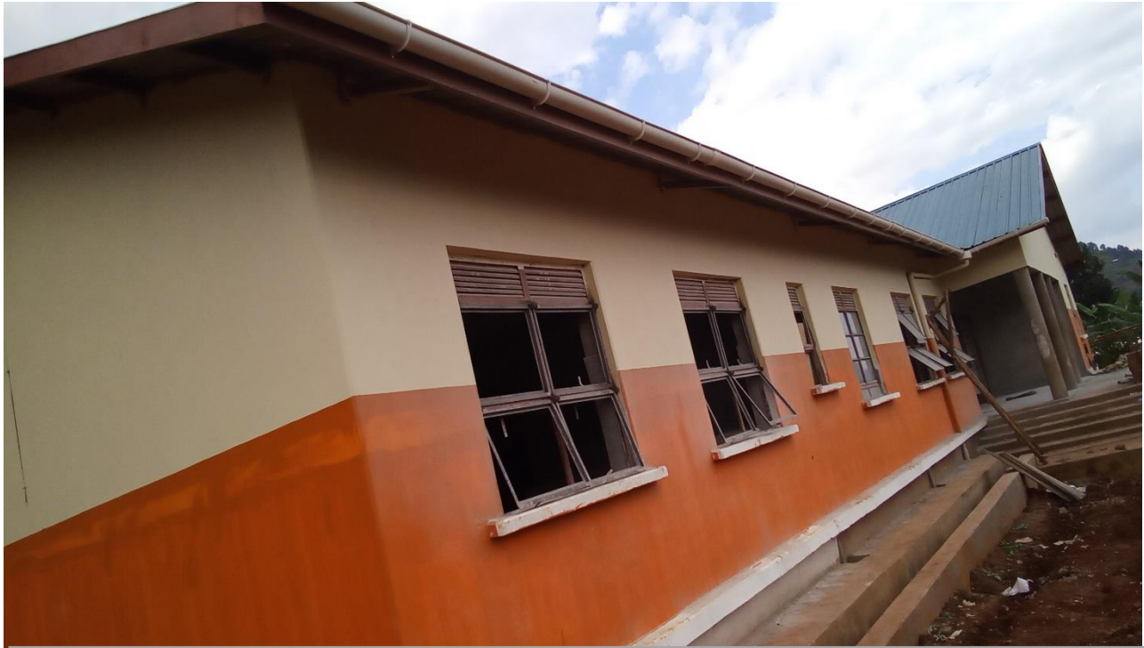
Maternity Ward at finishes at Bunamono Health Centre III
