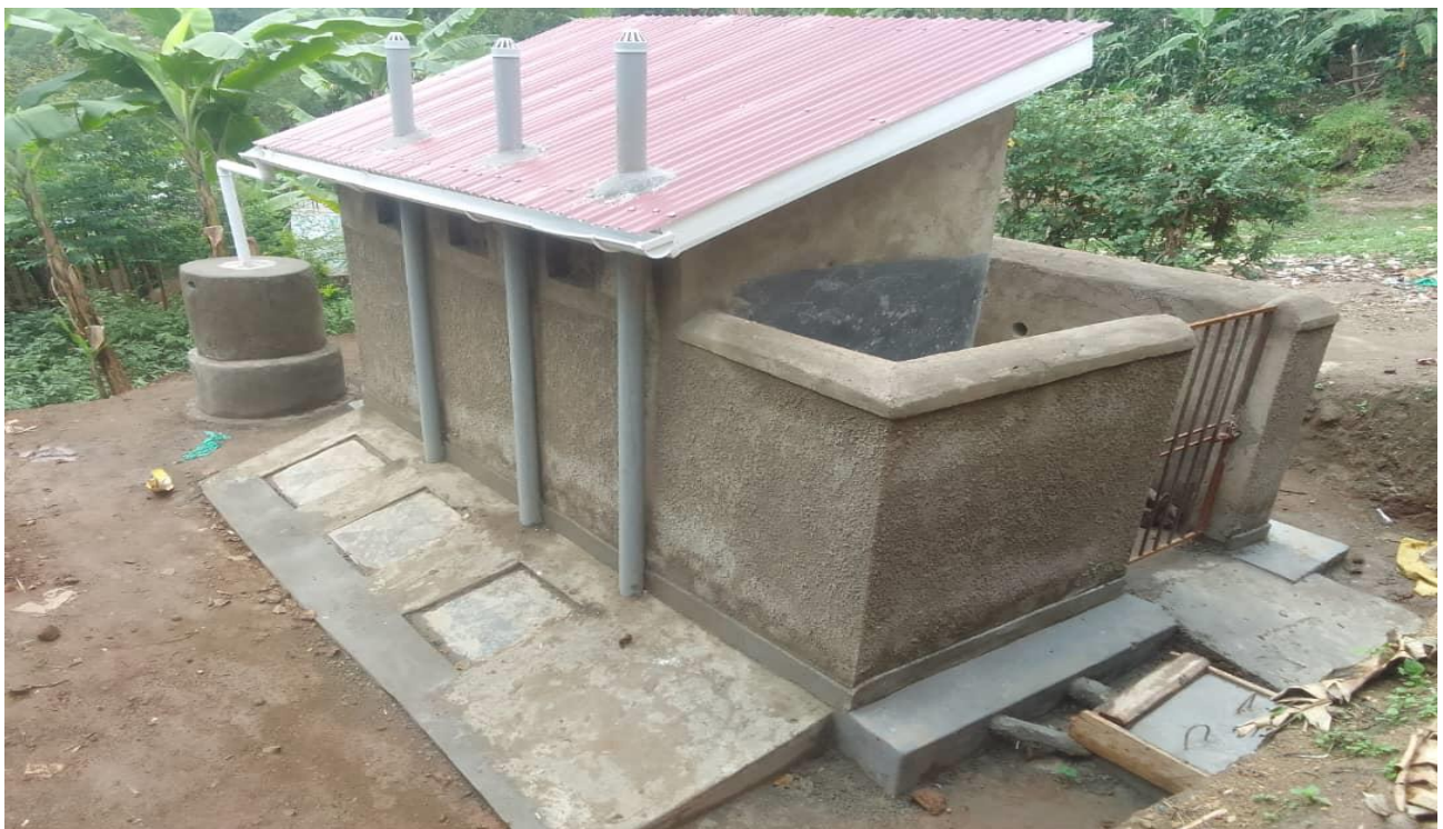
Itimbwa 3 stance composite latrine under construction
